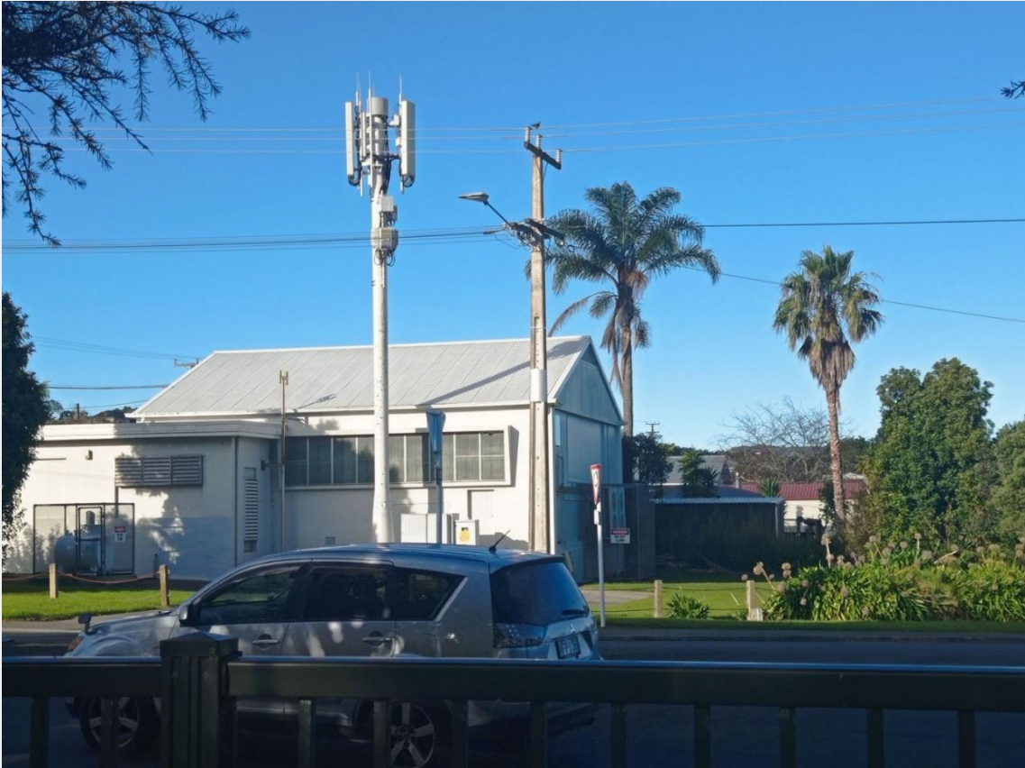
4G-5G mobile (macro-cell) cell tower only about 50 metres from the boundary fence of Onerahi Primary (Whangārei) – photo by author
