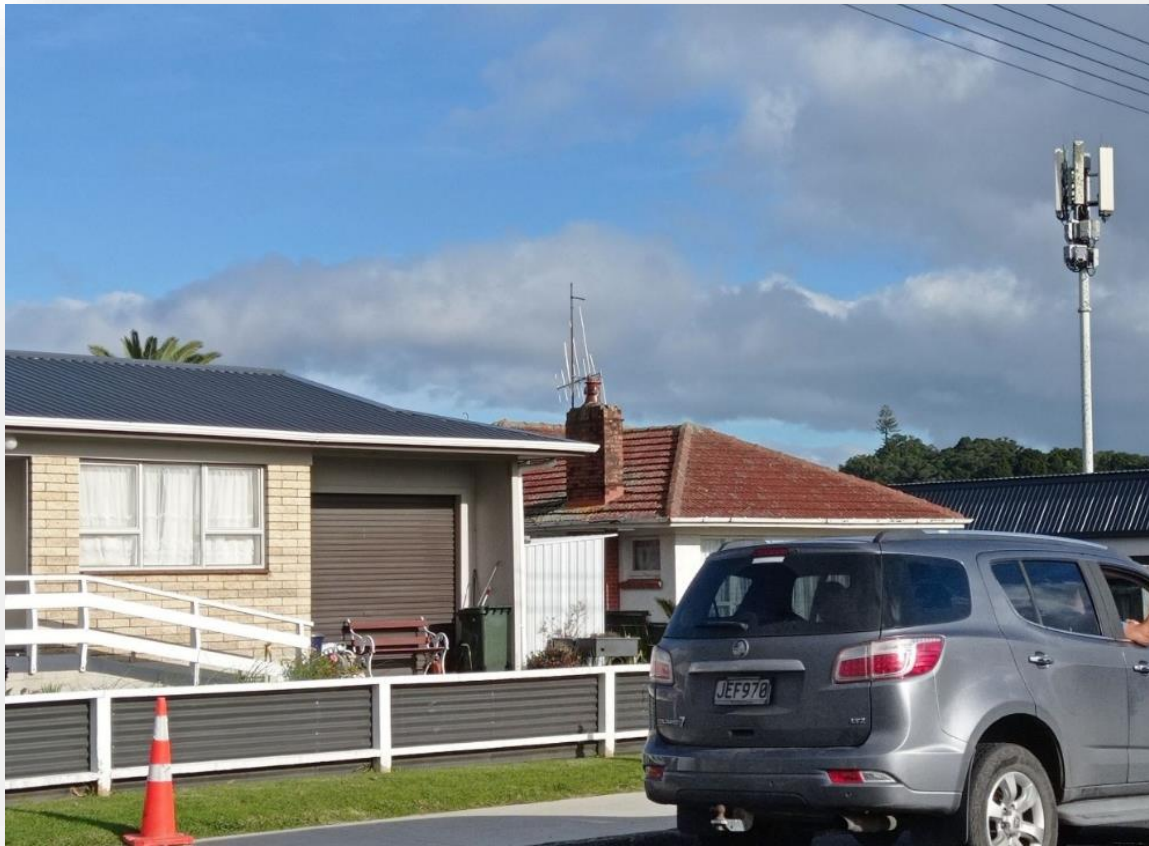
Kamo (Whangārei) – large (macro-cell) 4G-5G mobile cell tower less than 40 metres from residential housing – photo by author
