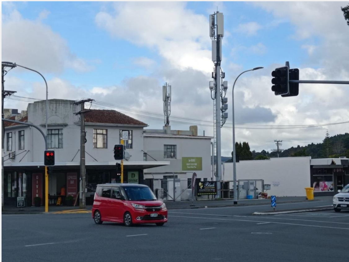
Kensington (Whangārei) Shopping Centre – 2 dominating large (macro-cell) mobile cell towers – photo by author
